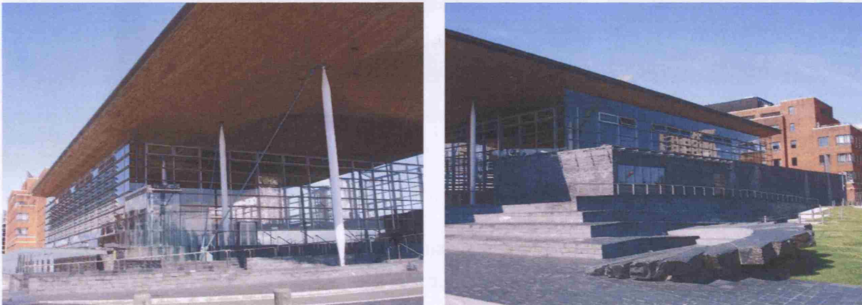
Figure 31: General form of the building observed from east and west side of the building (Source: photo by author)
