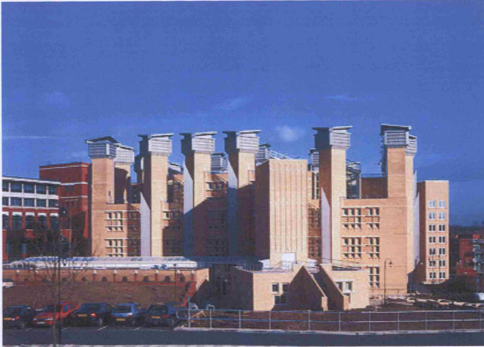
Figure 49: Main view of Lanchester Library (Source: Short and Associates)
