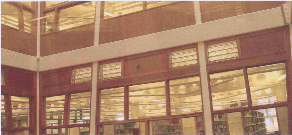
Figure 55: View of the central lightwell and the vents (Source: Cook et al.)
