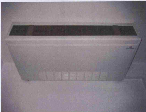
Figure 25: Room fan coils
