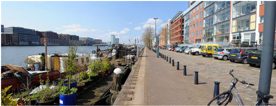
Image 8.5 - Java Island Urban Development, Amsterdam, The Netherlands (1990-2000); Masterplan: Sjoerd Soeters Office; Client: Municipality of Amsterdam.
