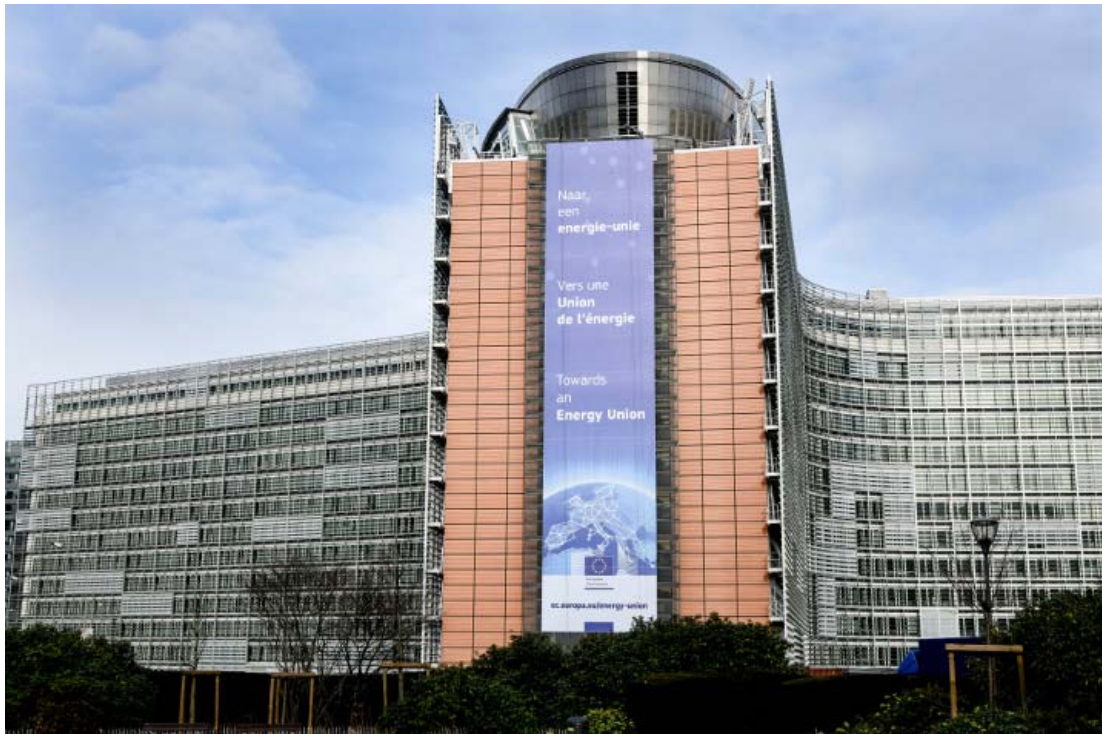
Image 6.1 – Berlaymont building, Headquarters of the European Commission, Brussels, Belgium (1975; rebuilt in 2004); Architect: Lucien De Vestel with Jean Gilson; Client: EC; Image: EC.
