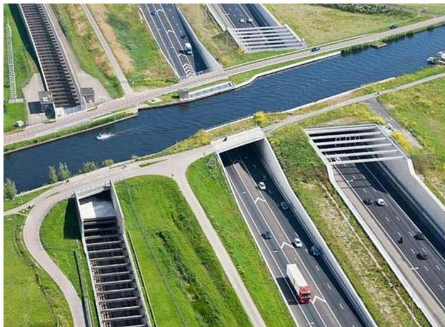
Image 8.11 – Aqueduct Ringvaart over the A4 Highway, Haarlemmermeer, The Netherlands (2006).
