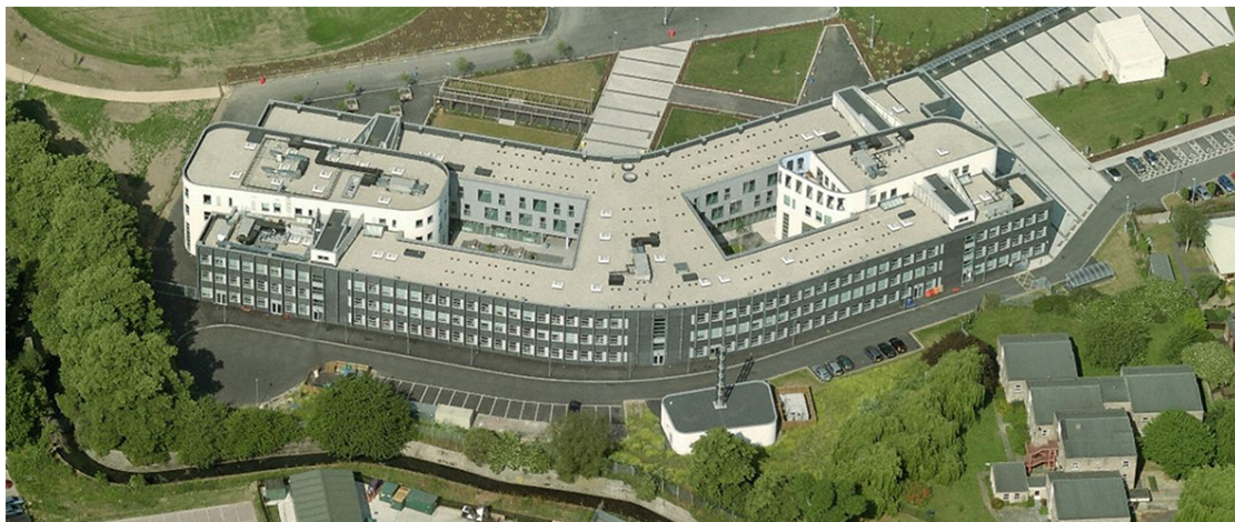
Figure 8.3: Loxford School: aerial satellite view
