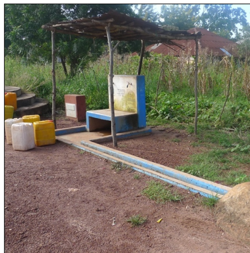
Figure 29. Standpipe with shade
