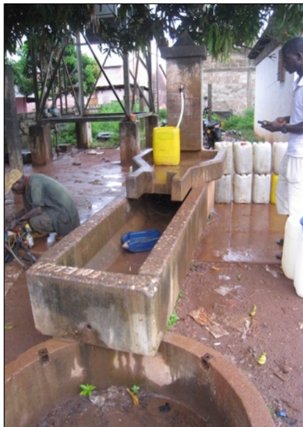
Figure 11. The one standpipe in operation in 2006 (picture taken in 2010)
