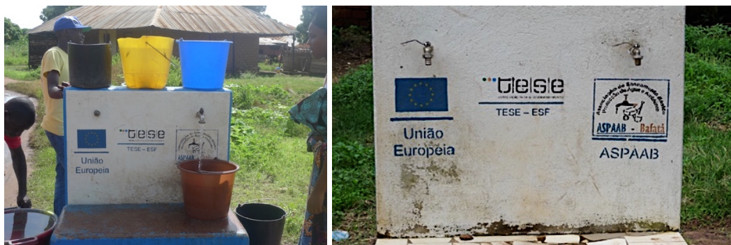
Figure 10. Standpipes in Bafatá (pictures taken by myself in 2014)
