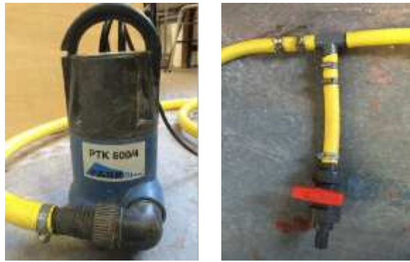
Figure 47 Submersible pump and control valve installed to regulate the recirculated flow
