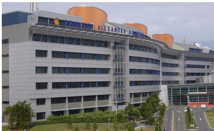
Figure A.5 Princess Alexandra Hospital in England with Solar thermal collectors (Princess Alexandra Hospital, n.d.)
