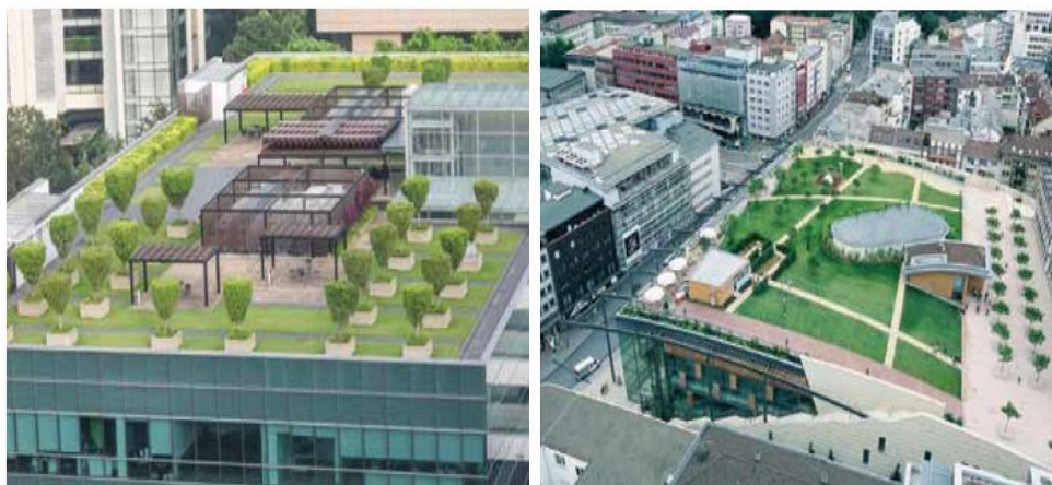
Figure A.15 Examples of extensive and intensive green roofs Left: Extensive green roof Right: Intensive green roof (Source: Hui, 2013)
