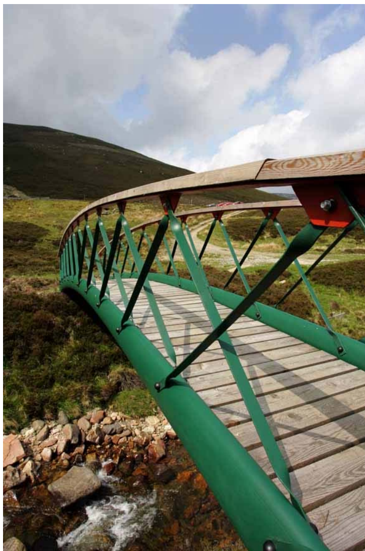
Fig. 2. Society Bridge, Scotland (2005)
