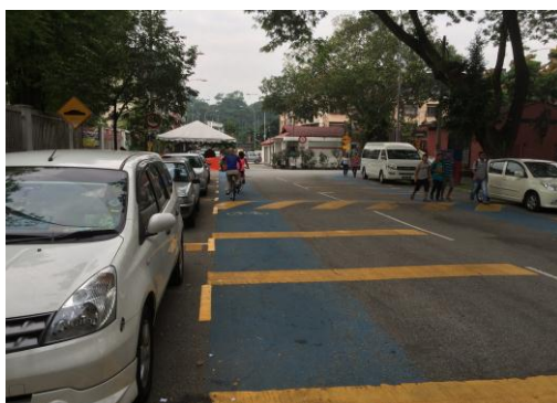
Fig. 9. Problems with the new cycling pathway in KL in Brickfields area: (a) a bike pathway is “squeezed” between on-street parking and traffic (left); (b) not enough space is left for cars to drive through between the two newly introduced bike pathways (right).
