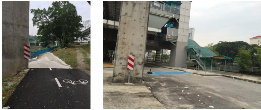
Fig. 12. Inadequate clearance on the cycling pathway, just before Brickfields area, it is difficult to find the route to continue your journey.
