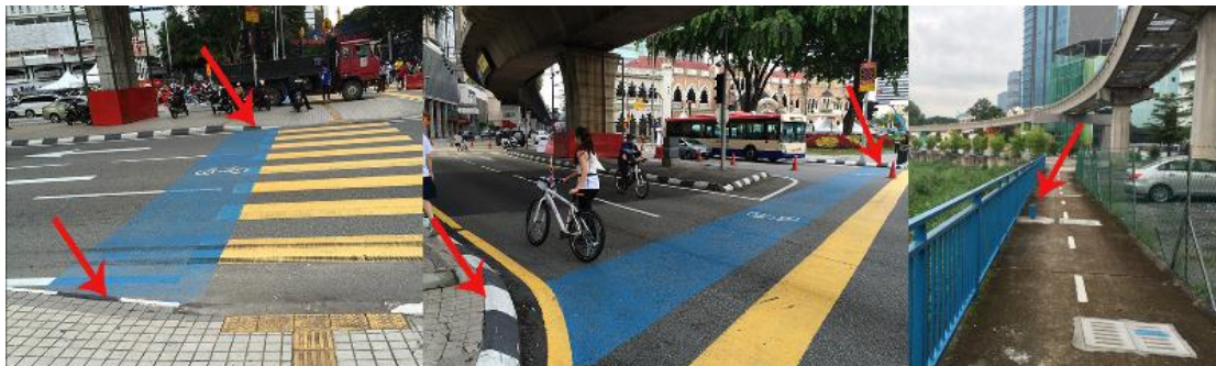
Fig. 11. Problems with the new cycling pathway in KL in front of the city hall and along the river: (a) designated cycling pathway at intersection that force cyclists to hop the curb (left); (b) obstacles in the middle of the cycling pathway that can potentially put cyclists at risk if two cyclists have to pass by each other.
