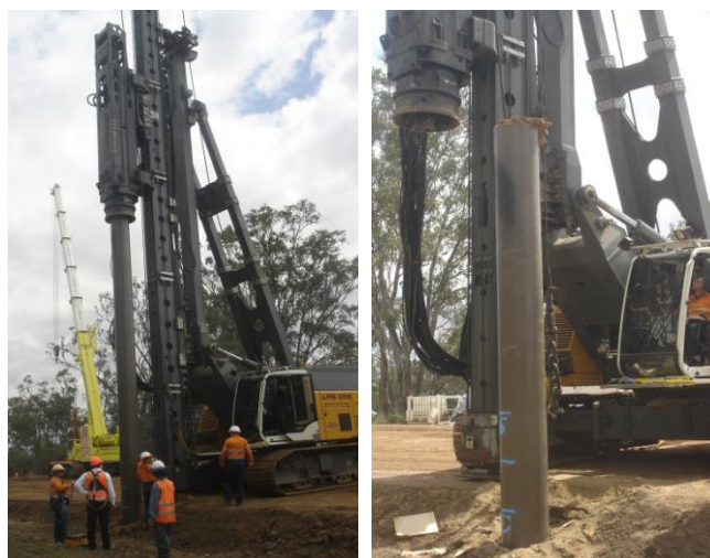
FIGURE 02: Pile driving rig for trial test.
