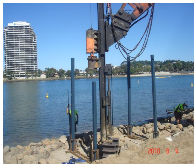
FIGURE 01: Application of composite pile.
