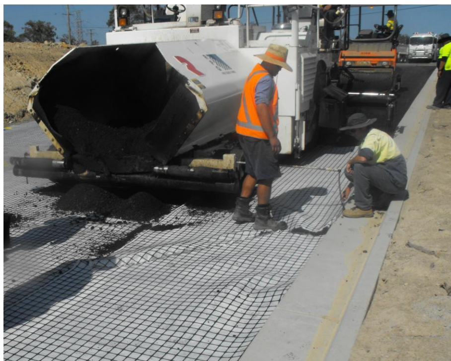
Figure 8.6 Rippling affect during placement of the Tensar ARG Asphalt Reinforcement Grid
