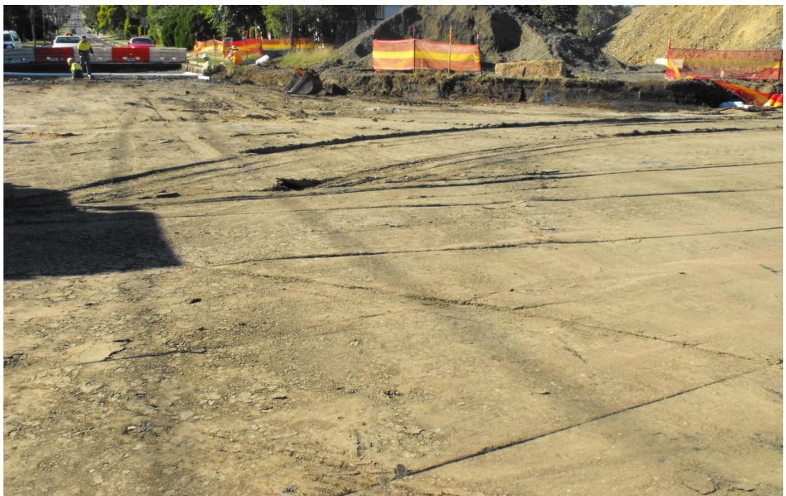
Figure 8.9 Subgrade surface following a proof roll with a laden water truck
