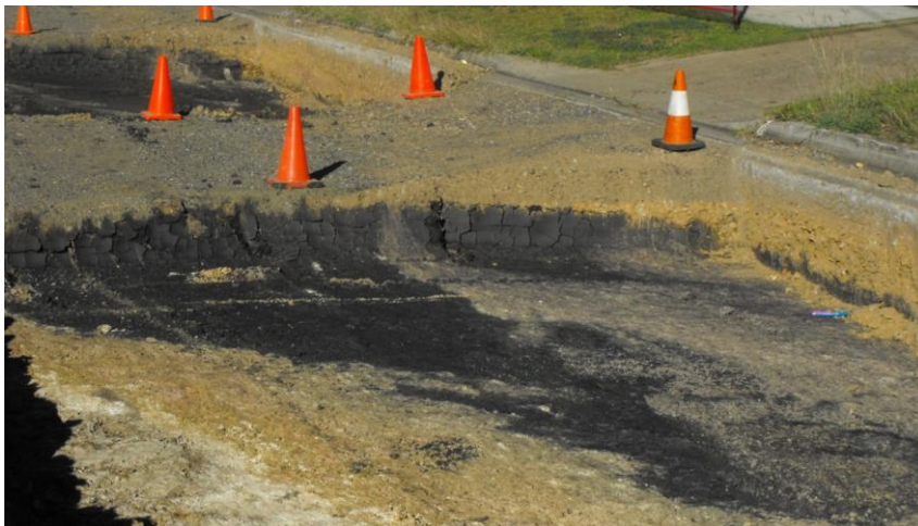
Figure 8.7 Blacksoil on Whitehill Rd
