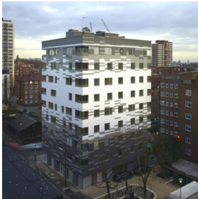
Figure 2.1: Stadhaus Building, London 2010 ( Tall Timber Buildings The Stadhaus, Hoxton, London 2010 )
