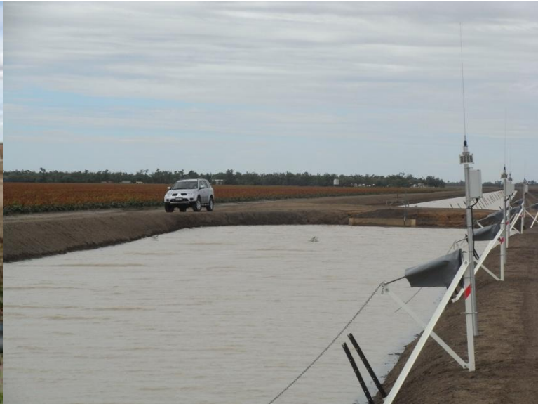
Figure 2. Automated (PTBs) for furrow irrigation.
