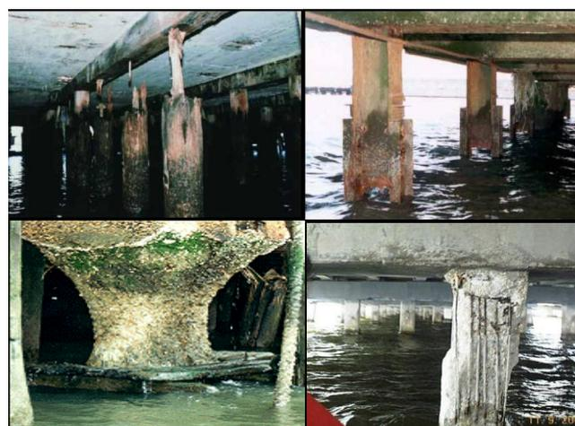
Figure 1. Degradation of traditional piles [3 & 4].
