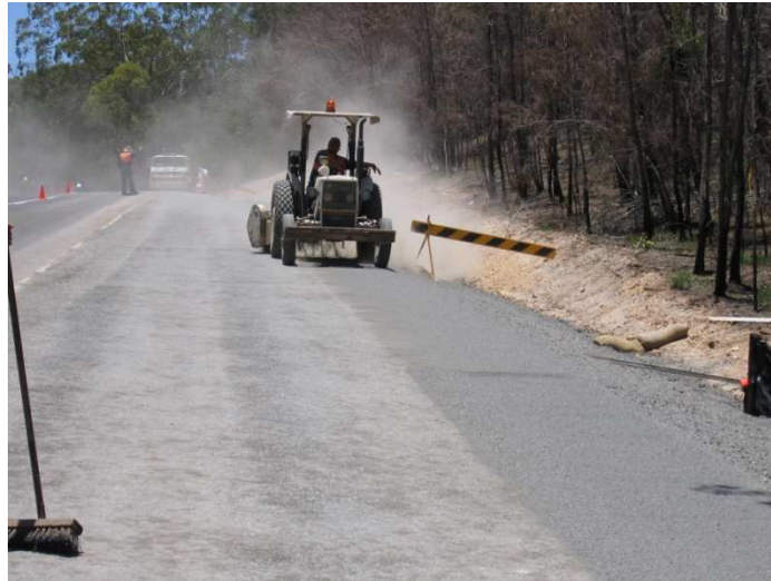
(8) Figure 2.3.1.1 – Sweeping the surface in preparation for spraying bitumen
