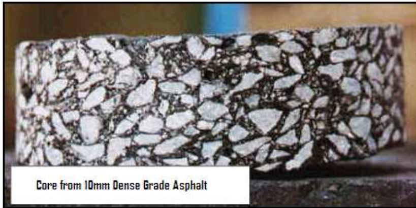
(4) Figure 2.4.1 – Core sample of dense graded asphalt
