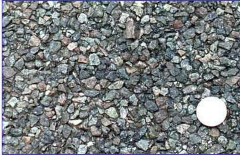
(3) Figure 2.5.1 – Typical 10mm chip seal surface
