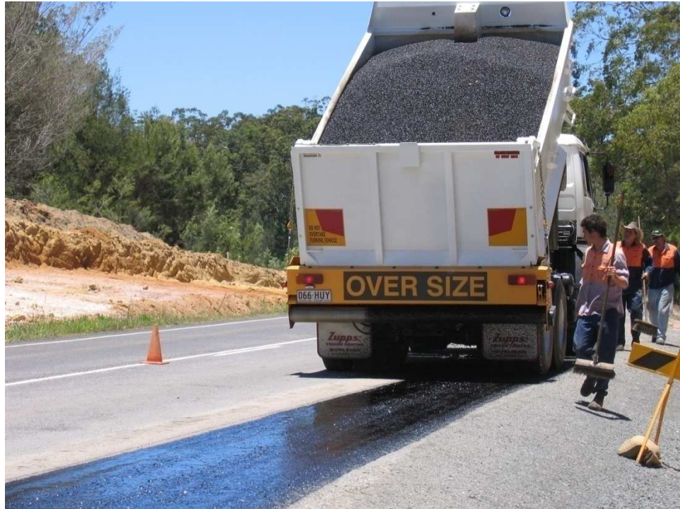
(9) Figure 2.3.2.1 – Aggregate spreading onto sprayed bitumen
