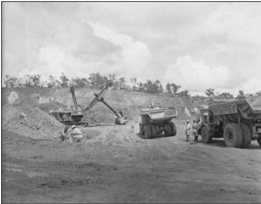
B. 5 Dysons Open Cut 1958 taken from Archives of Australia
