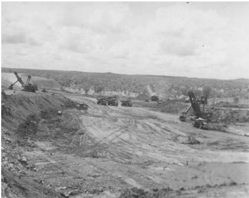
B. 6 Dysons Open Cut 1958 taken from Archives of Australia
