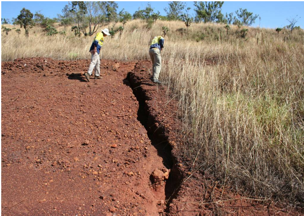
B. 7 Dysons landform, evidence of monsoonal scour at site of maximum settlement, April 2008
