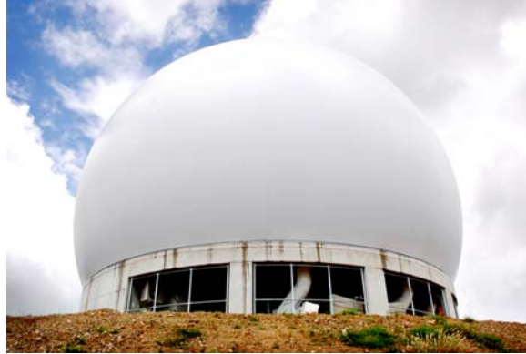
Figure 4.4. CP2 site infrastructure at Redbank Plains. Antenna and pedestal are within an inflated radome mounted over housing for office, storage and transceiver.
