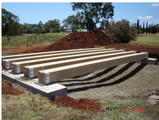
Figure 1 Hybrid Composite Bridge Beams
