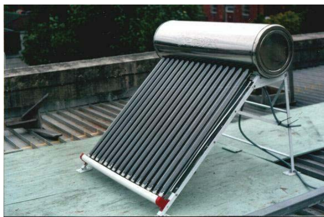
Fig. 1 The evacuated-tube thermal solar collector.
