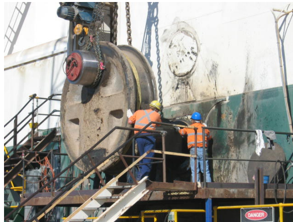
Fig. 6.6 Propel eccentric mechanism being dismantled on shutdown.
