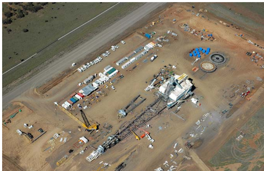
Fig. 3.3 Aerial view - Dragline shutdown site.
