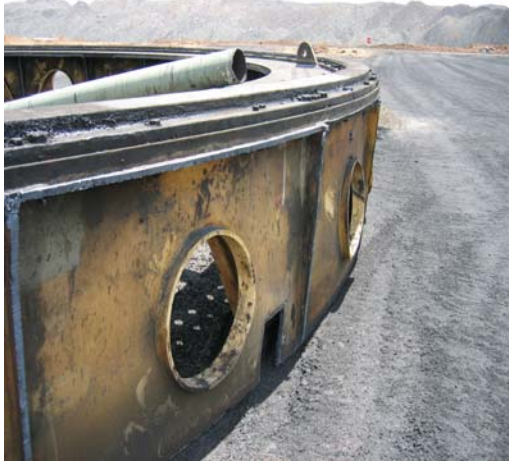
Fig. 6.1a Double diaphragm removed during a major shutdown
