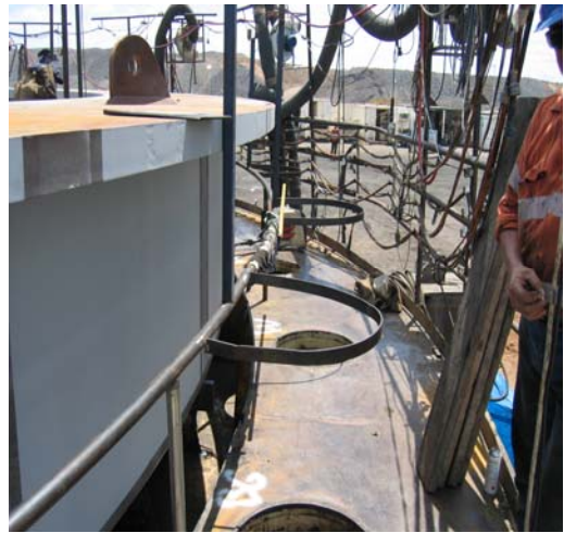
Fig. 6.1b Single diaphragm section being installed into tub
