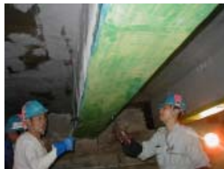
Fig. 6 Strengthening of beam
