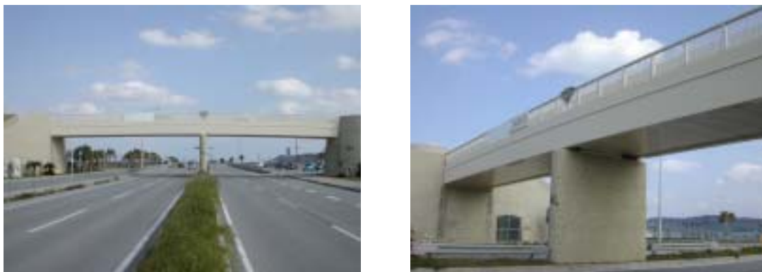
Figure 13 All FRP Pedestrian Bridge in Okinawa made of GFRP
