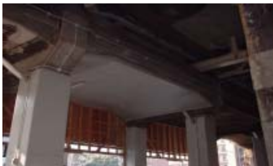
Fig. 5 Strengthening of slab
