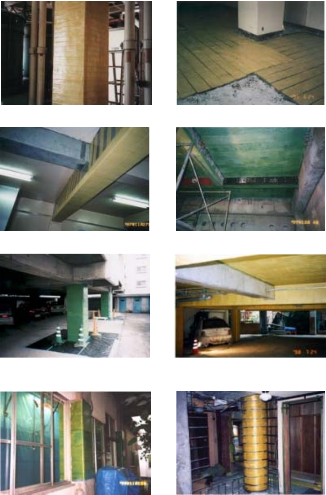
Fig. 7 Application of AFRP sheets in building structures
