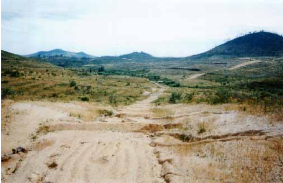
Figure 3. Cross-bars constructed on Old Pipeline Road
