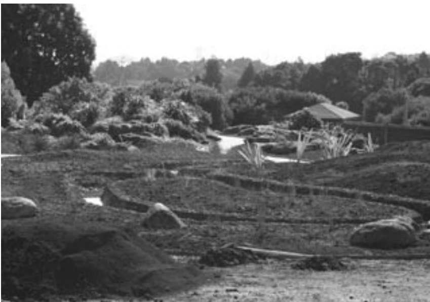
The construction of a replicated saline wetland habitat. Photo: Jack Hobbs
