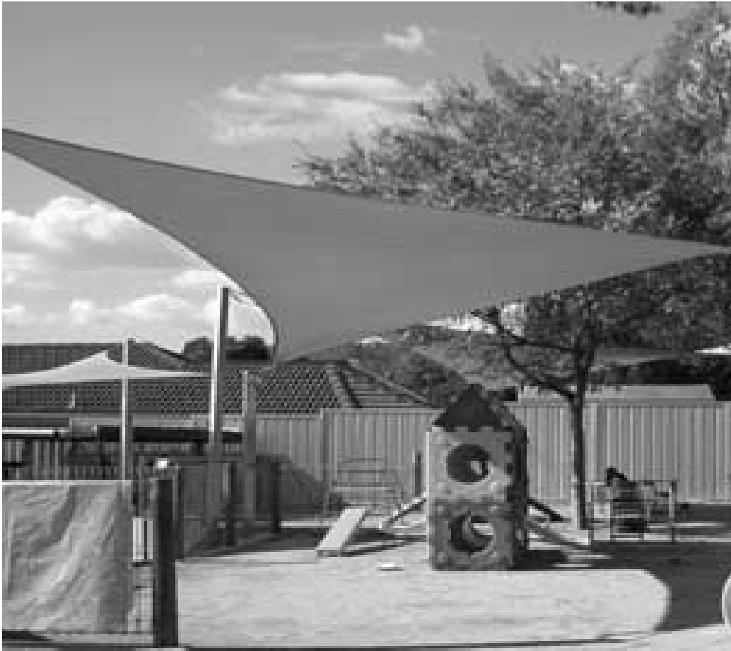
Figure 7.14. Shade sail used to cover play equipment.
