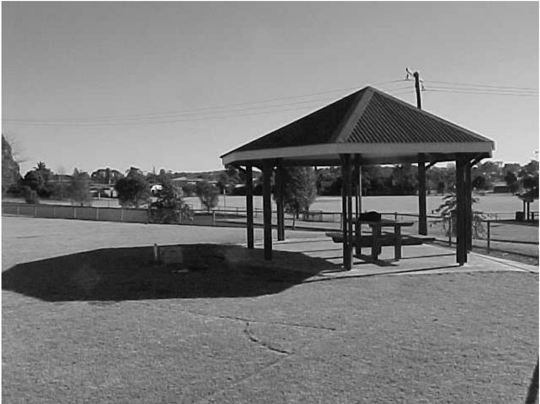
Figure 7.10. Large shade structure located at a sports field.
