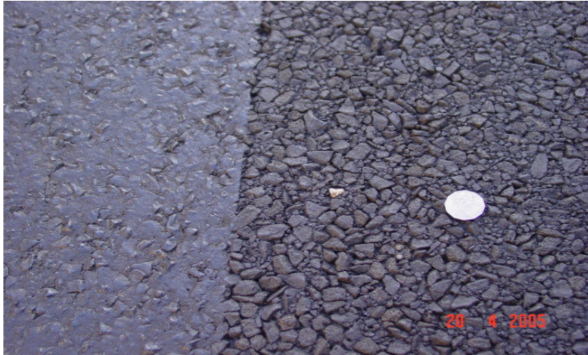
Figure 2.4 Results of High Pressure Washing (Source: Main Roads, Emerald)
