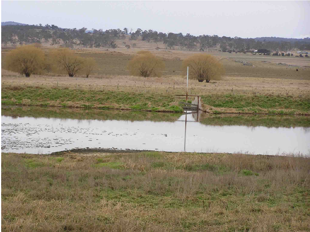
Figure 3.14: Feedlot B - North-East Sedimentation Basin Prior to Inflow
