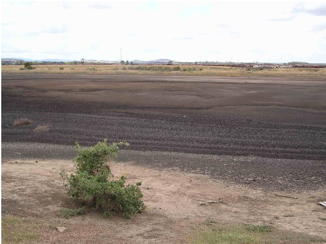
Figure 3.10: Feedlot A - Primary Holding Pond Primary to Inflow
