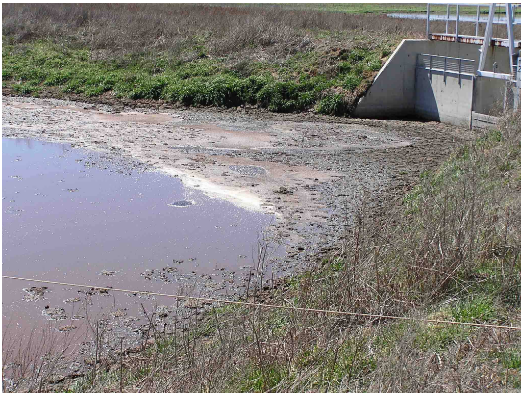
Figure 3.15: Feedlot B - South-East Sedimentation Basin Prior to Inflow
