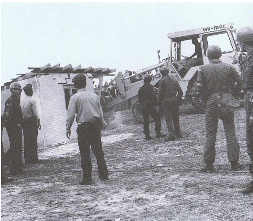
89 Bulldozeraktion in Küçükköy, August 1975
