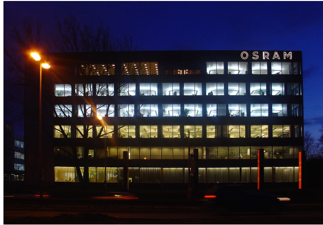
FIGURE 2.4. The OSRAM GmbH Headquarters in Munich, Germany during the study: in the top three floors, the illumination was changed to a blue-enriched light environment (LUMILUX SKYWHITE), while the lower ones remained with their initial lightning over the course of the study period.
