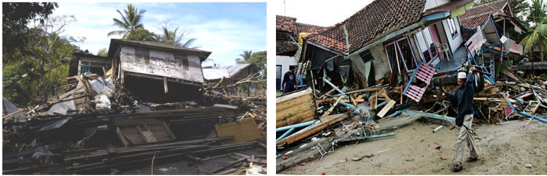
Figure 7.2. Typical small buildings which are vulnerable to tsunami hazard
