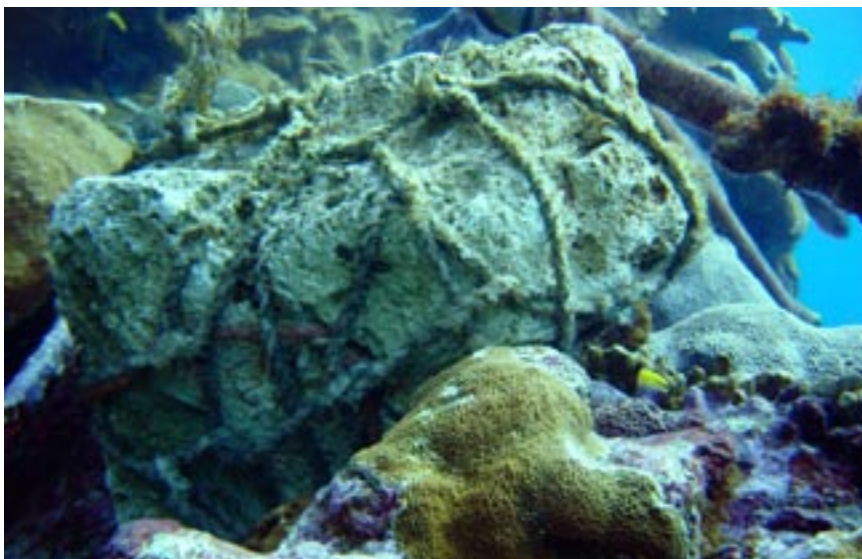
Figure 2.—Rock anchor in Lulu Bay used in temporary mooring system for fishing boats.
