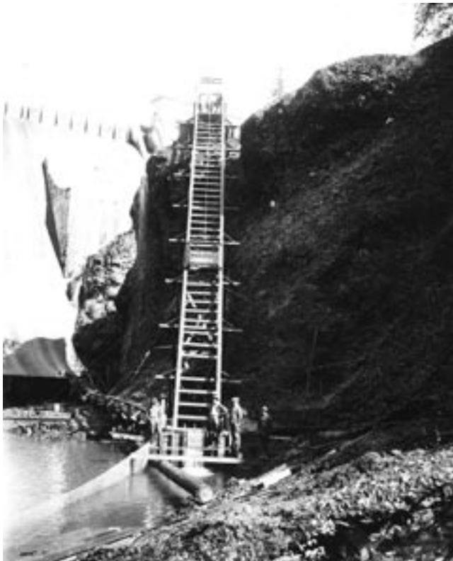
Figure 9.—Fish hoist [ca. 1924]. University of Washington Archives, John N. Cobb photographs, Collection no. 418, Box 5, Folder 183, print no. 5010.
