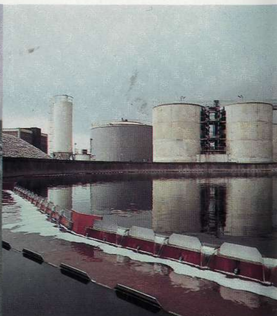
4.3 Clay Mills sewage works.
