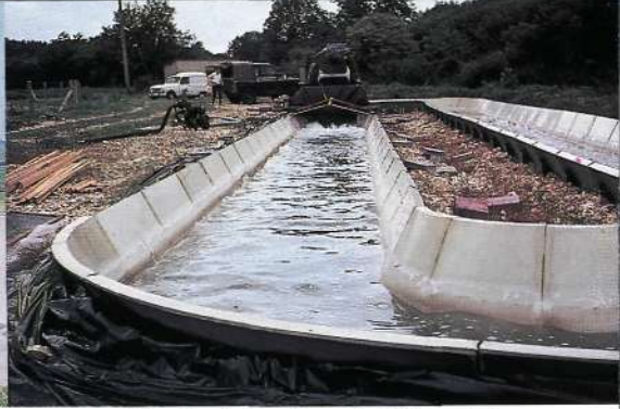
7.3 The circulating channel at Waterston.
