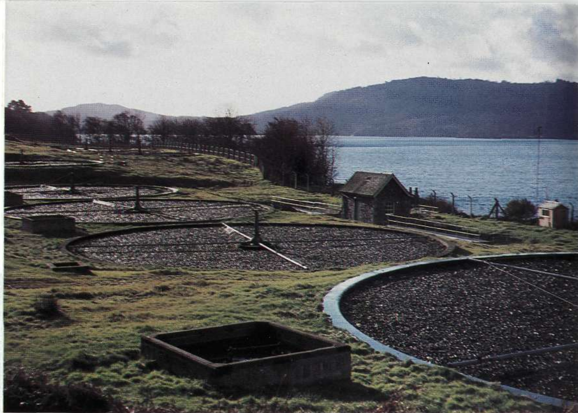
4.1 Windermere sewage works: trickling filters.
