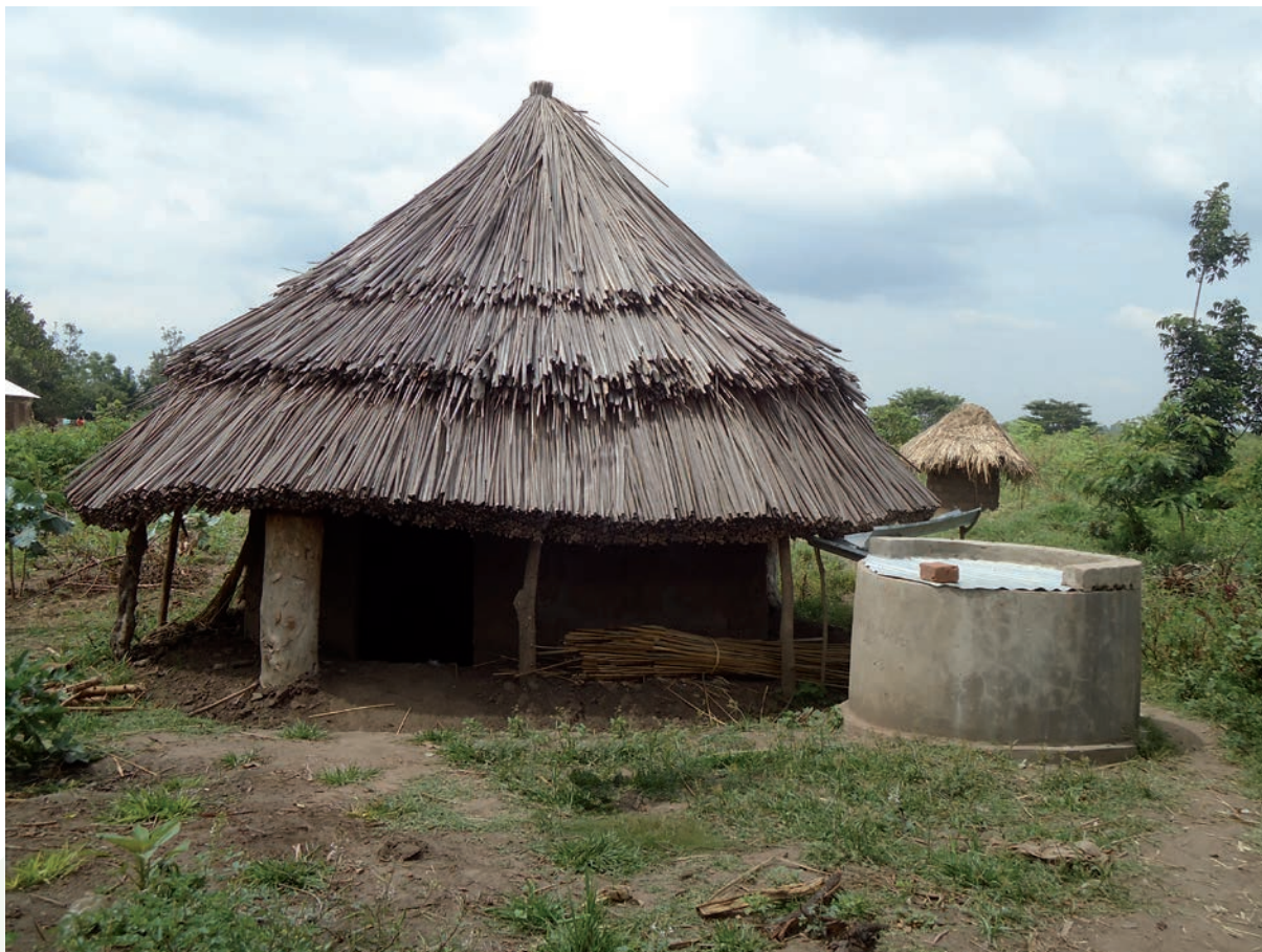
Above: Rain water is harvested from papyrus roof and stored in concrete tanks for use during periods of scarcity
