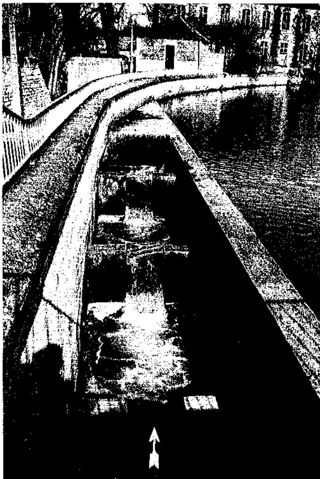
Figure 29 Two views of the completed 'pool and traverse' fish pass (arrowed) based on plans in Figure 28, showing detail inside the pass and its relation to an adjoining weir and radial sluice gate.
