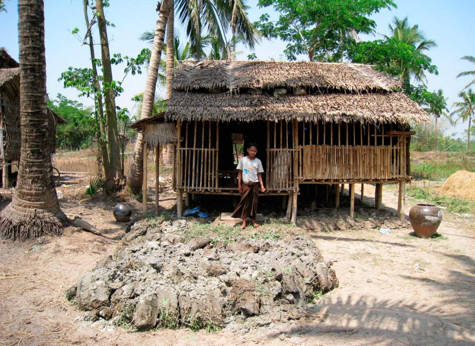
Excavated soil from the borrow pit being used to raise the level surrounding a house in Dedanaw village.
