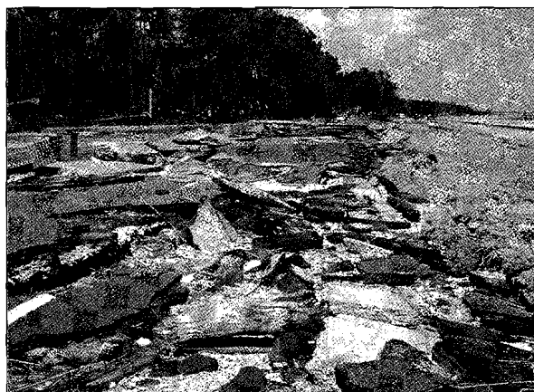
Shaped and battered by nature: Mississippi coast after Hurricane Camille, August 1969 (photo: NOAA).
