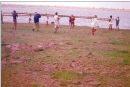
Figure 6. Installation of frame
