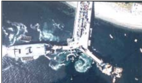
Vegetation near this commercial ferry in Washington State is impacted by shading and propeller wash associated with the dock.
