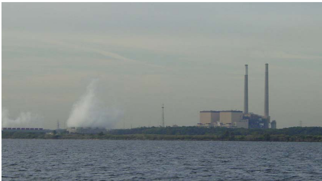
Baltimore power plant
