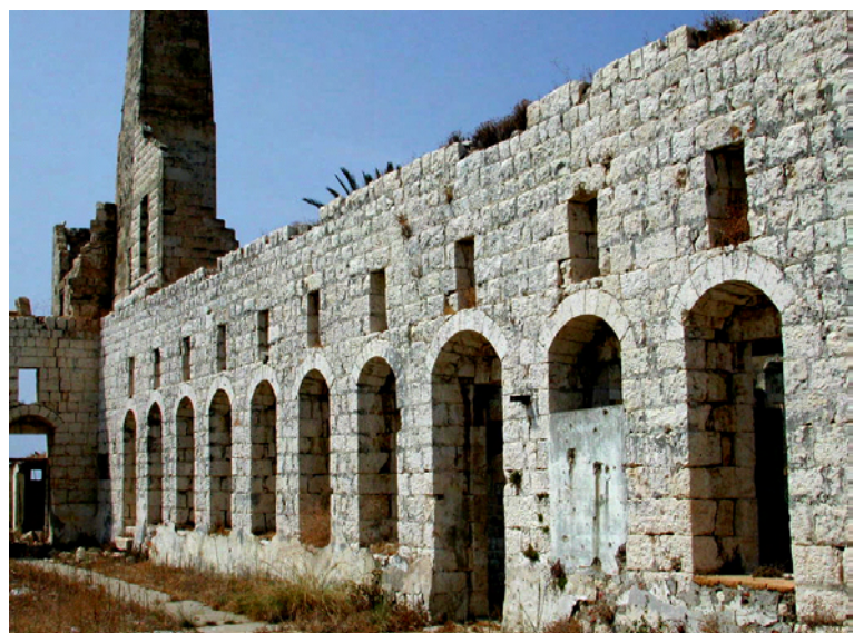
Photo 68: Remains of silk factory at Damour. The building maintains the links with the town's important industrial past
