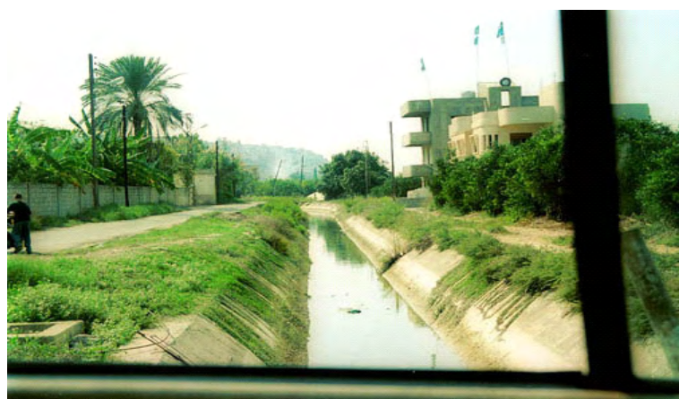
Photo 46: Irrigation channel, Sarafand (Litani project)
