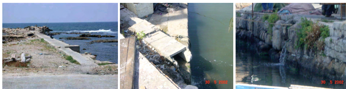
Photo 42, Photo 43, Photo 44: Outfalls and channels discharging wastewater directly into the sea in Sour
