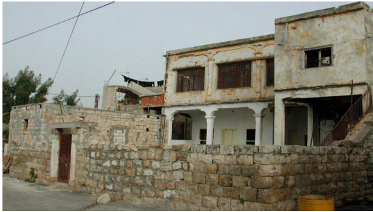
Photo 73: The old town core in Naqoura has potential for rehabilitation and re-adaptation
