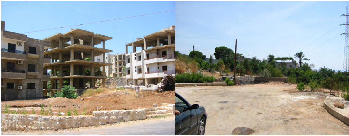
Photo 13, Photo 14: Examples of construction works
