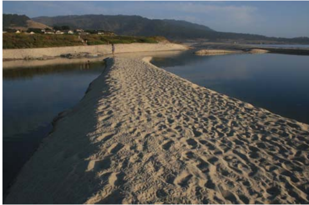
a. Lagoon outflow was restricted at the 2005 breach site with the help of a dozer and sandbags. (17 Jul. 2006)
