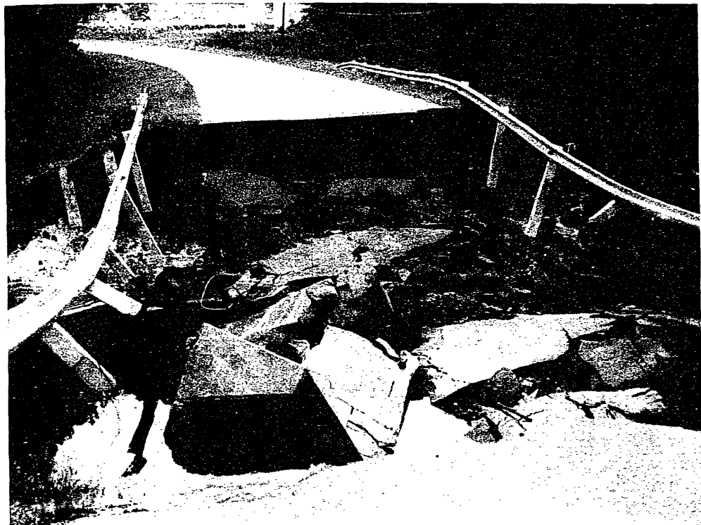
Figure 22.—Salem Branch at State Highway 159 near Havana.
