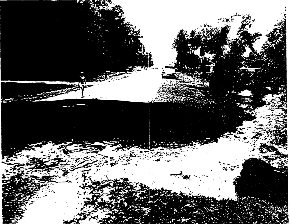
Figure 21.—Road washout at North Lake Drive between Old Bainbridge Road and Lake Jackson—Photo by Tallahassee Democrat.
