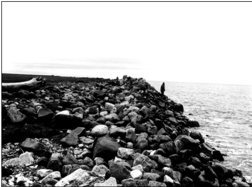
Figure 6. Photos of the Camden Bay, Alaska boulder ridge (from Barnes 1982).
