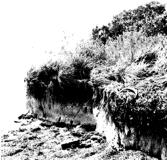
Figure 10. A section of the Flamingo Embankment (Craighead, 1971) along northern shores of Florida Bay near Flamingo, Everglades National Park.
