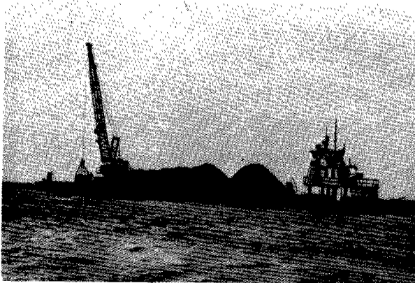
Figure 3. Shell barges, crane barge, and towboat for planting shell.
