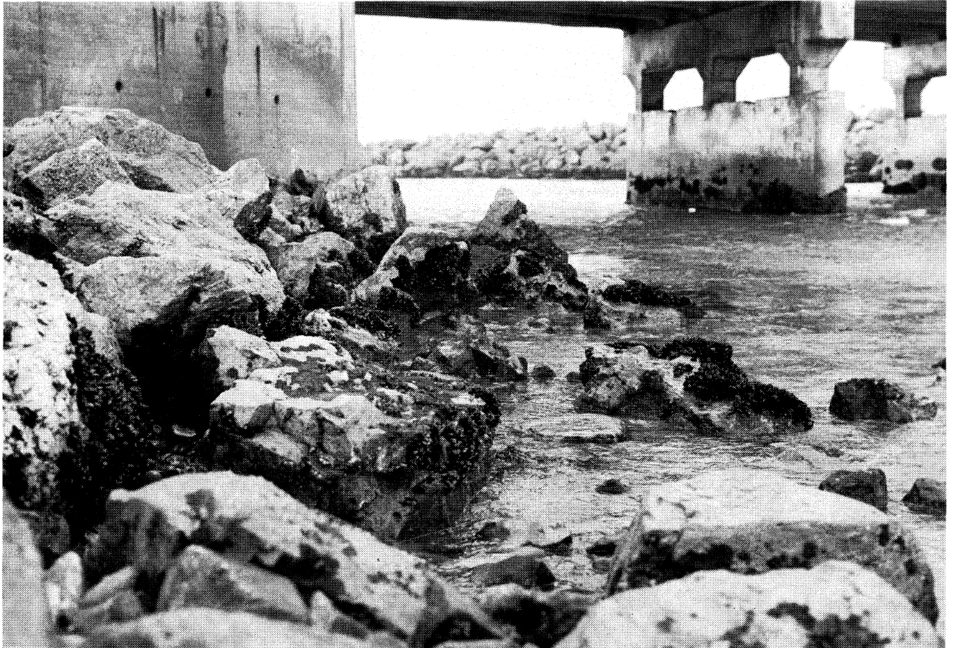
Dredging the lagoon to create an adequate tidal prism, ensures cooling waters for the power plant, and has also created a healthy marine ecosystem.
