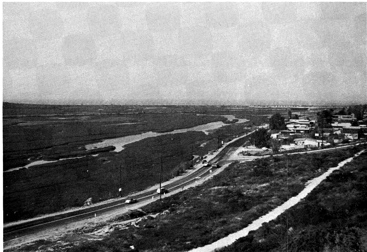
Top Photo: The Santa Fe Railroad right-of-way is a dominant feature and reduces the vitality and aesthetic quality of the lagoon.
