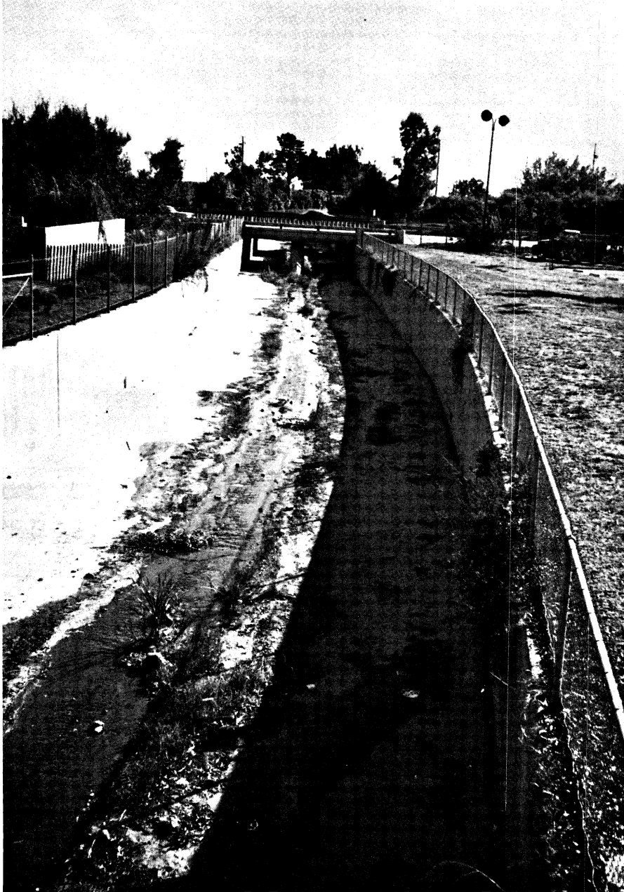
Completion of the Carpinteria Watershed Project should greatly reduce existing flood control and sedimentation problems in the marsh.
