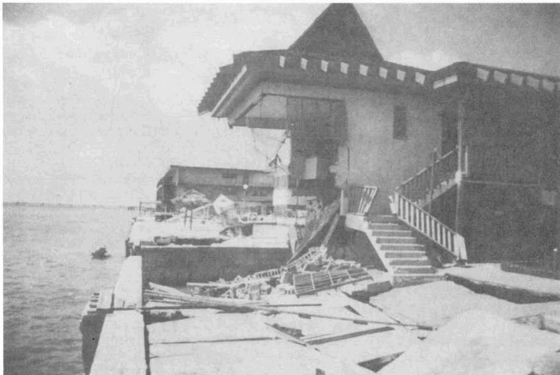
Figure 15. Hurricane Elena (1985) damage (From Clark, 1986a).
