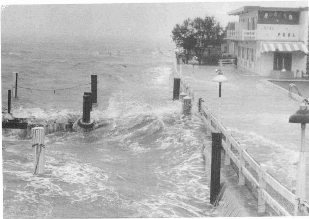
Figure 8. Hurricane Donna. Even though Hurricane Donna did not strike Miami, this photograph shows typical damage along Dade County shoreline (Courtesy of National Hurricane Center).
