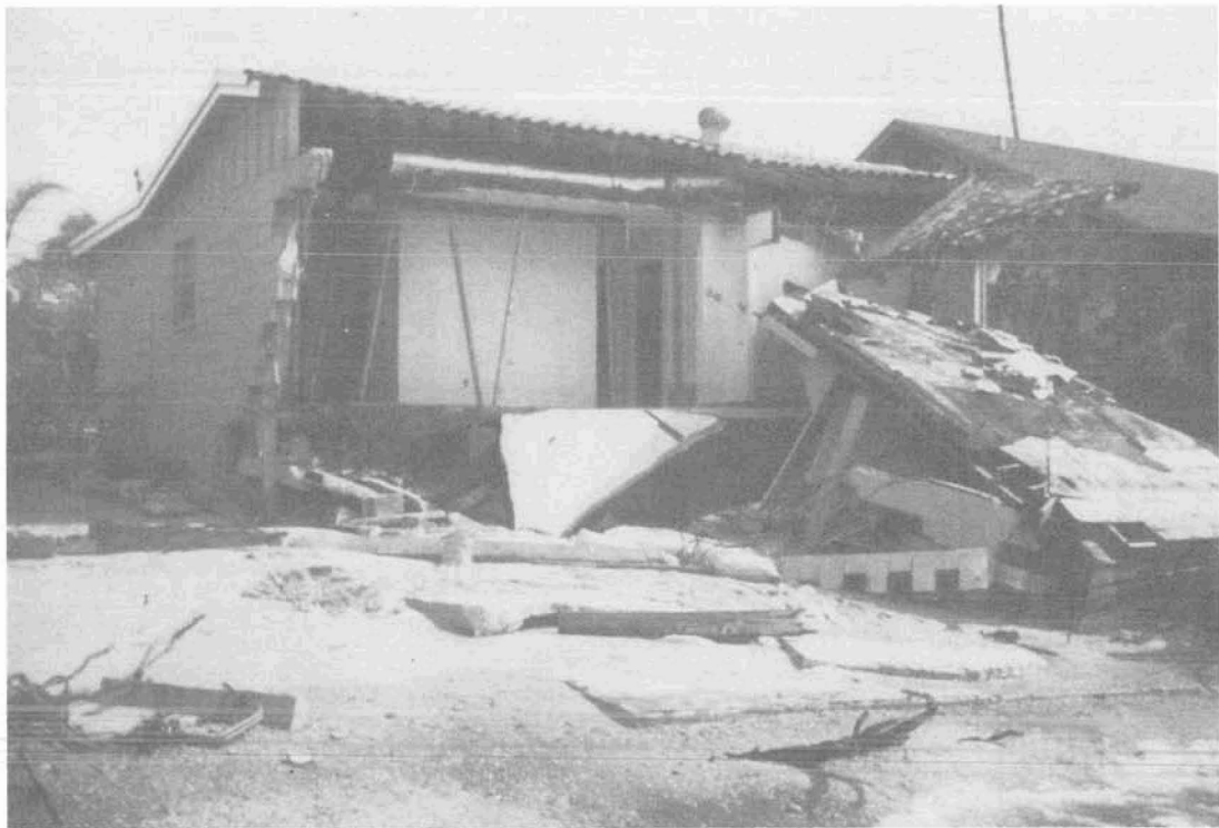
Figure 16a. Hurricane Juan (1985) damage (From Clark, 1986a).
