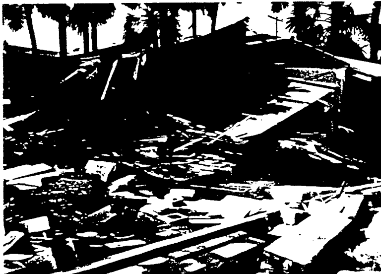
Figure 7: Structure With Foundation On Grade Totally Demolished By Wave Force.
