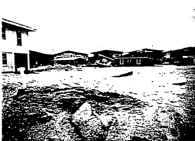
Figure 5: Sand Washover on Second Row of Houses (North of Waccamaw Avenue, Garden City).
