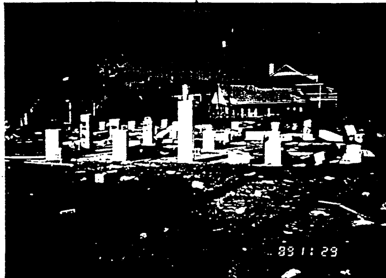
Figure 11: Masonry Pier Made of Concrete Blocks Failed Due to Weak Joint and Inadequate Fill.
