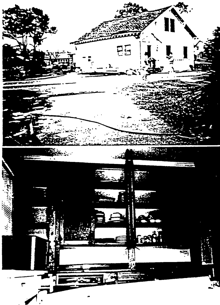
Figure 8: (a) Structure Built On Slab Floated Away From Foundation And Deposited 100 Feet Away Across the Street. (b) The Arrangement Inside the Kitchen Remained Undisturbed in the House.
