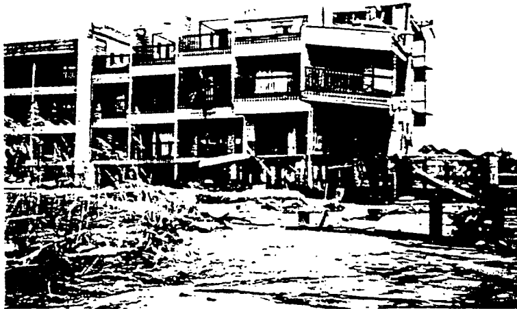
Figure 15: (a) Modular Unit Constructions With Poor Connections
