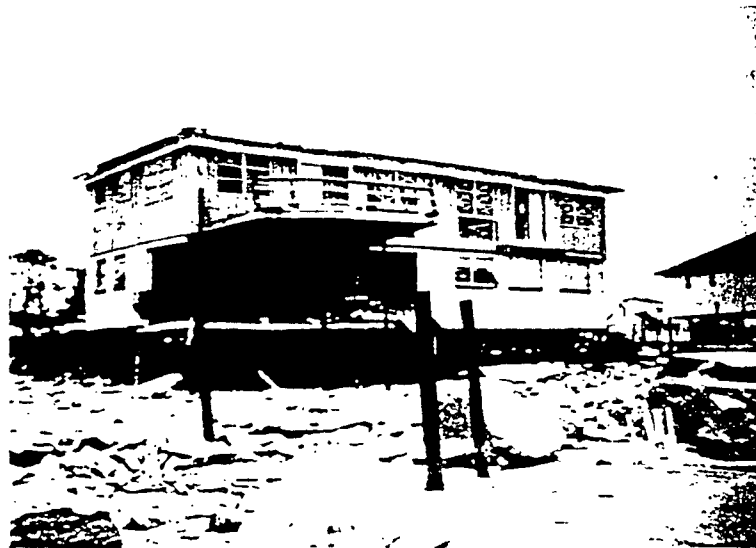
Figure 14: (b) The Access Ramp Washed Into the House Due to Wave Force.
